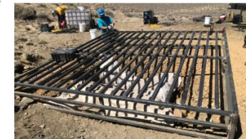
Finishing a bat cupola over a shaft with tarps protecting the timber below
