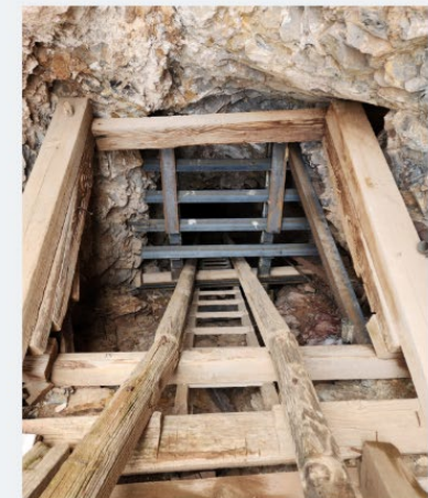
Before and after safeguarding steep mine entry in Death Valley National Park, Inyo County, California
